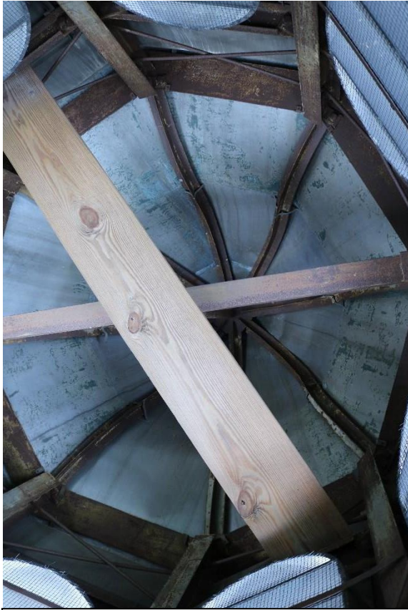
Cupola wood framing and metal work (2021 photo)
